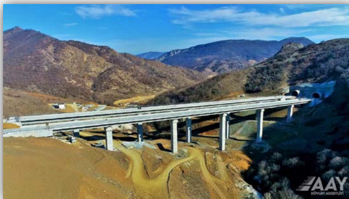
Construction of Ahmadbayli-Fuzuli-Shusha road is in full swing. Source: < http://www.aayda.gov.az/ >, February 2023.
